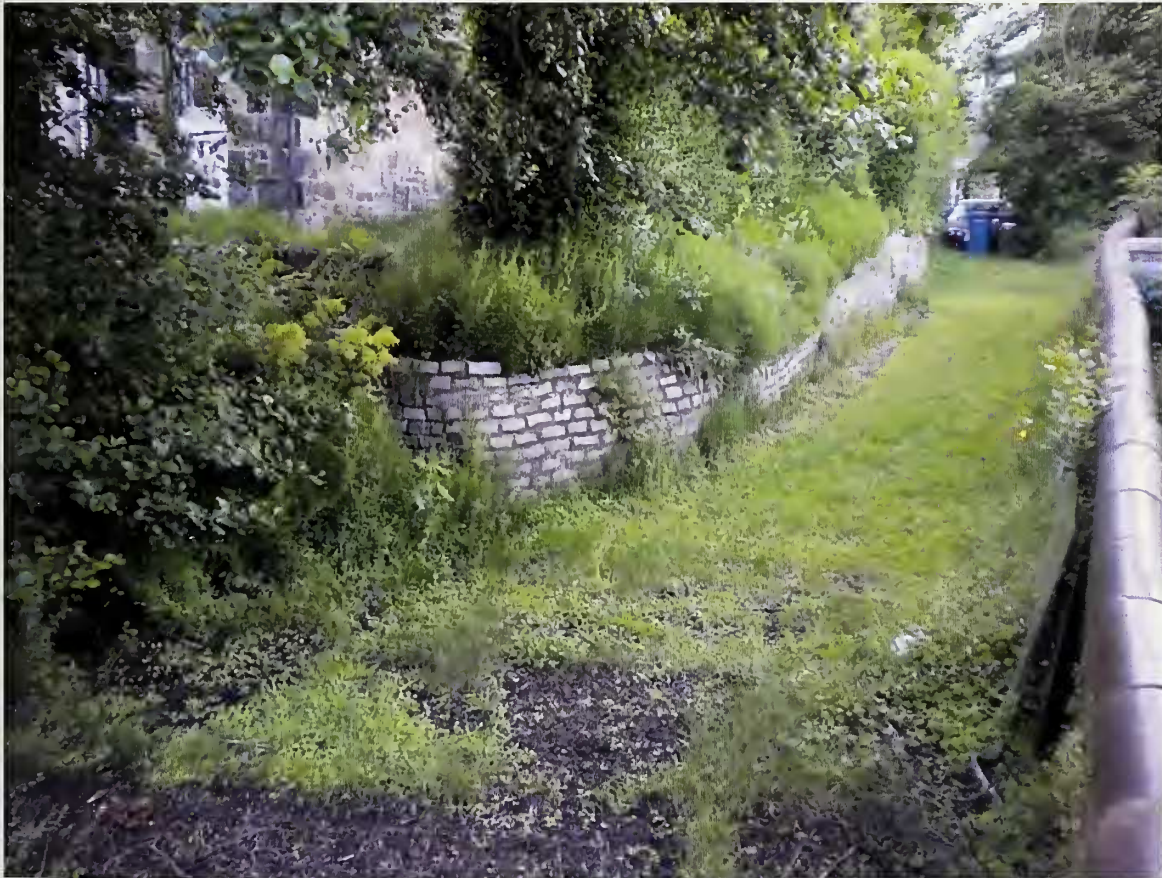
Fig.2. Newark Drive - Grassed over concrete driveway.
